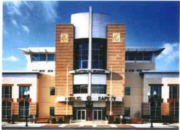
Clayton C. Graham Public Safety Building Atlantic City, NJ
